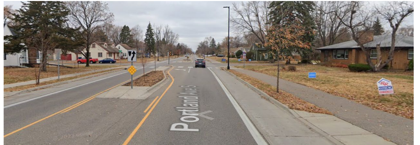
2022 Shared use path Concrete shoulders Crossing islands
