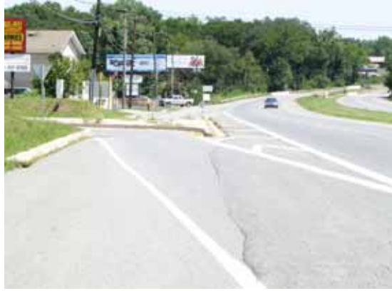
Pavement striping fronting the channelization island on US 40, near Sycamore Drive, interferes with bicycle traffic.
