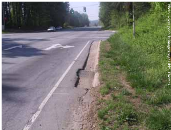
Broken pavement in the shoulder is unsafe and uninviting to bicyclists.
