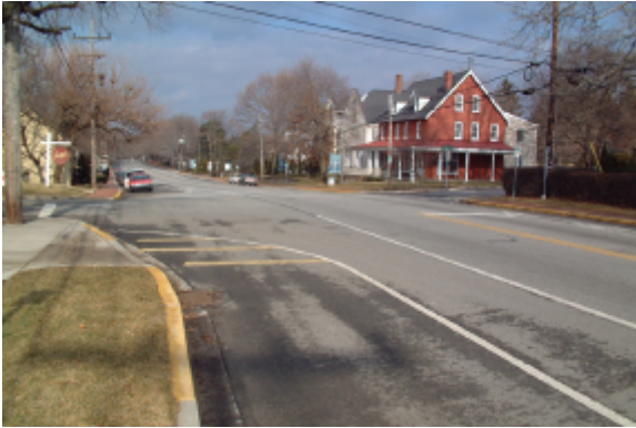
7T - Existing Condition Looking North
