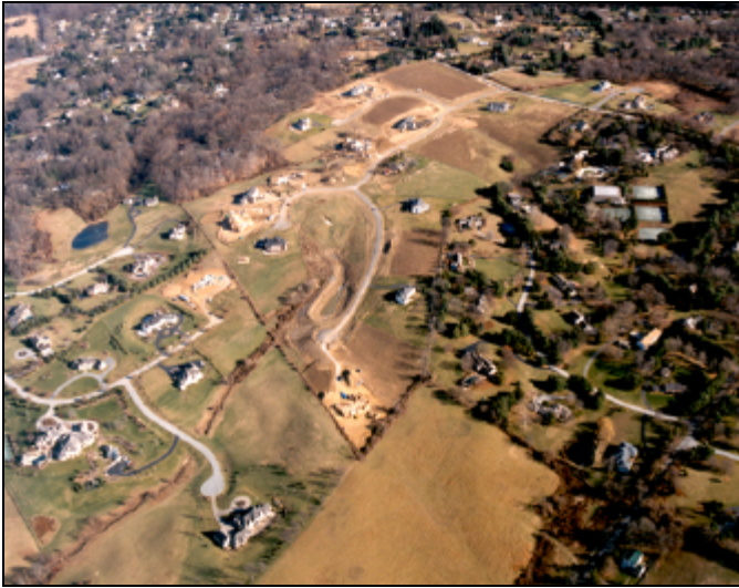
2A - Aerial View of Large Lot Subdivision Development
