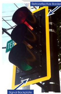
Figure 4-7: Backplate with Retroreflective Border (Source: FHWA)
