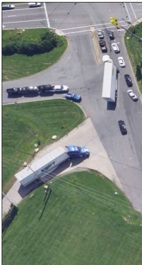
Figure 4-9: Intersection of Belle Hill Road and Elkton Road (Source: Bing Maps)
