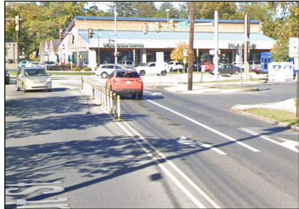
Figure 4-17: Example Left Turn Restriction at Service Station Driveway using Flexible Post Delineators (Source: Google Maps)
