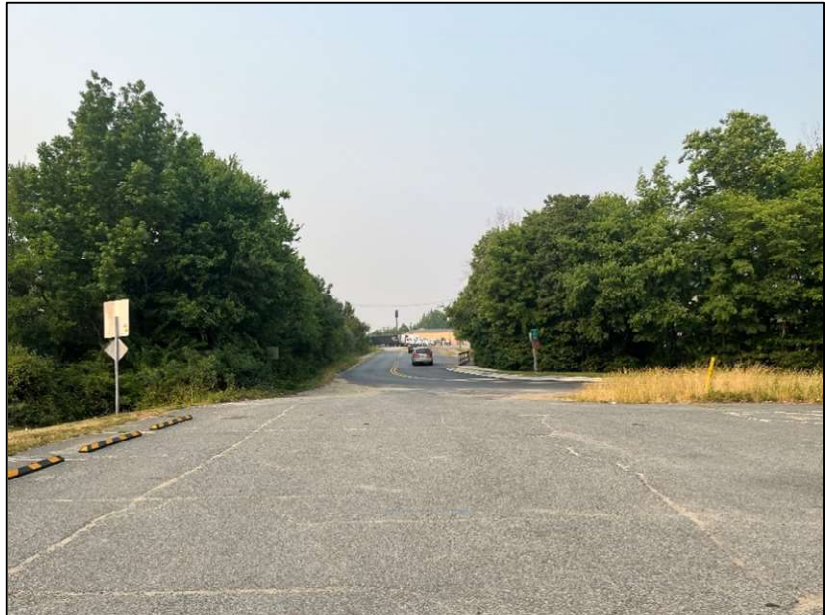
Figure 3-2: I-95 at MD 279 Park and Ride Facility
