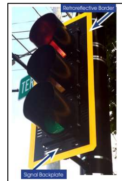
Figure 4-8: Backplate with Retroreflective Border (Source: FHWA)
