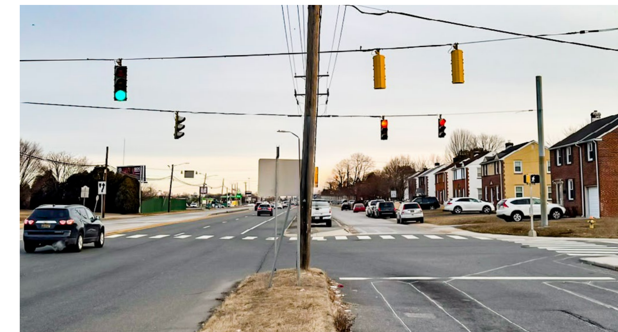
Example of Access Management, SR 9 North of New Castle
