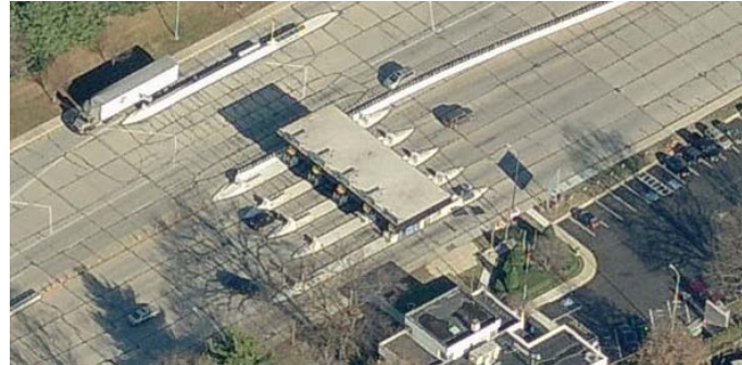
Tolling facility at the Hatem Bridge on US 40 (Source: Bing Maps)
