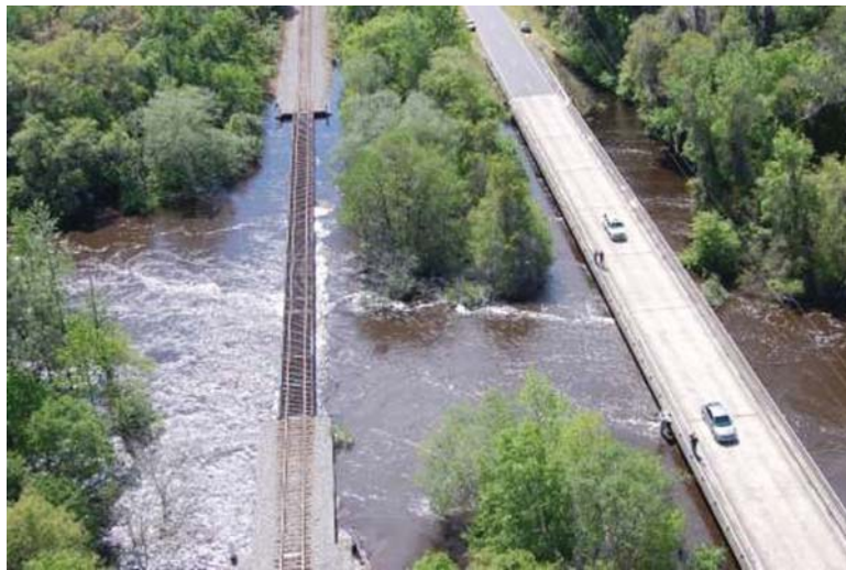
Flooding of State Route 141 due to Suwanee River Flood, Florida (Source: USGS)
