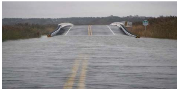
A Flooded Roadway on Route 9 at Appoquinimink River Bridge (Source: Delaware Coastal Programs)
