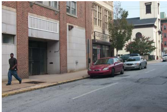
Concentrations of vacant, disbeveled or boarded up buildings can make pedestrians feel unsafe.
