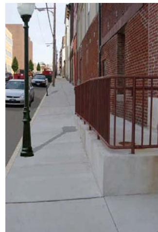
Desirable Condition (proposed) The existing ornamental railings behind Ships Tavern are aesthetically pleasing and reflect the building's architecture.
