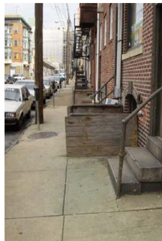
Undesirable Condition (existing) Pipe railings and plywood edges add to the visual clutter along the sidewalk between 7th and 8th Streets.
