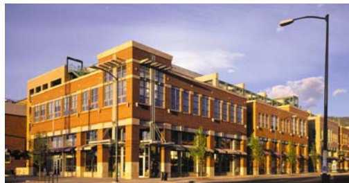
Retail wrapped around a parking structure.
