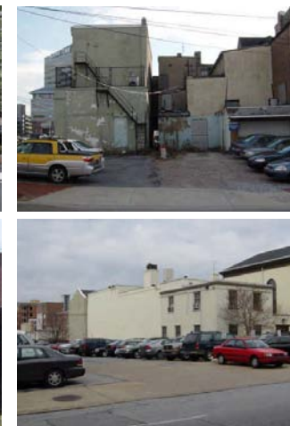
Undesirable Condition Having surface parking adjacent to the pedestrian sidewalk with no defined edge is not only aesthetically displeasing, but dangerous as well in instances where vehicles must cross the sidewalk.
