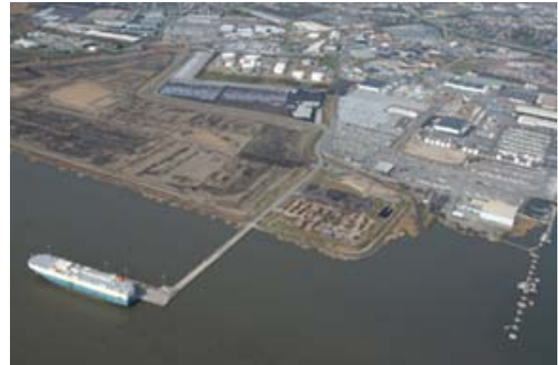
Photo courtesy of Port of Wilmington
