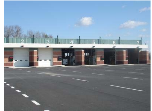
New Mid-County DMV will have a design similar to the Georgetown location shown above
