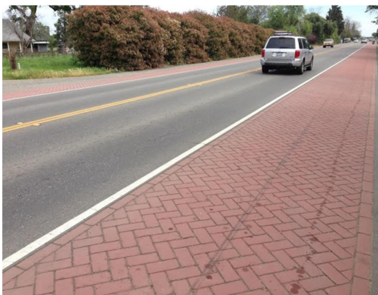
Shoulder markings and textured pavement can help calm traffic by narrowing the perceived width of a street (Source: Alta Planning and Design)
