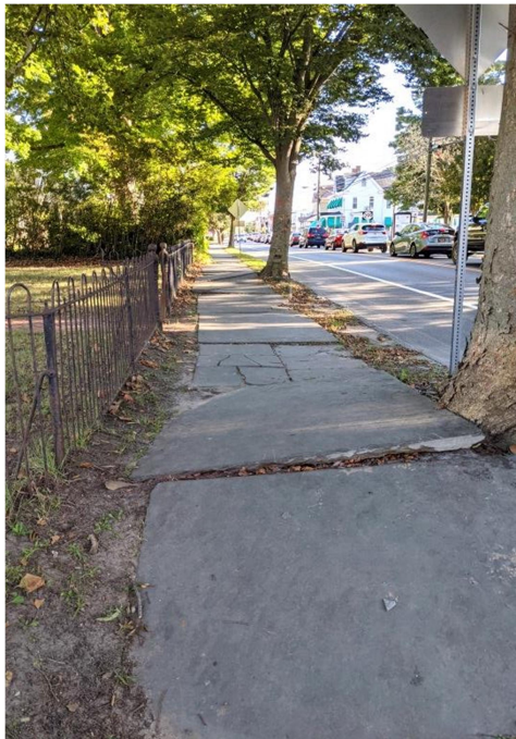
This section of sidewalk on the east side of Broad Street, just south of Lake Street, has been uplifted by tree roots.
