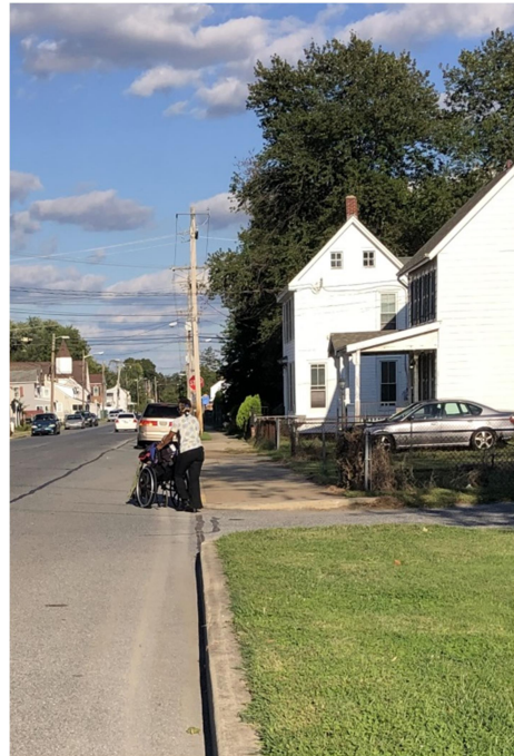
Sections of Lake Street lack sidewalks and curb ramps, forcing people with disabilities to move into the street.
