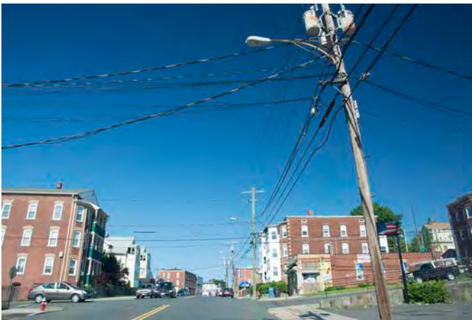
Overhead Utilities on Broad at Booth
