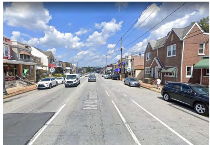
sample Wilmington streets: Orange St at 9th, Union St at 8th, Heald St at C Street
