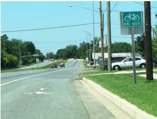
Along US 40, west of Landing Lane, bike signage and bike route pavement markings encourage usage.
