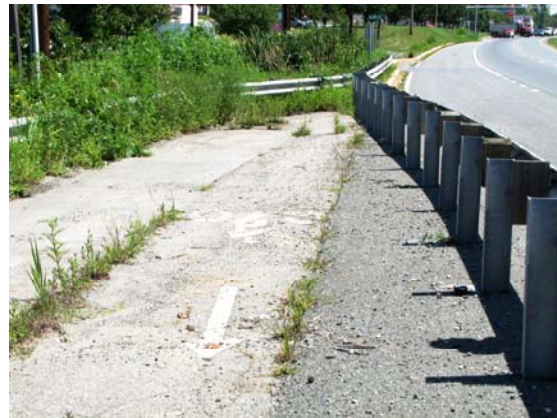
Along US 40, west of Mechanics Valley Rd., a shoulder with bike route pavement markings is inaccessible and forces bicyclists to use adjacent travel lane.
