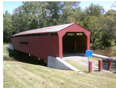
MD 272/ N. East Rd., Gilpin Falls Bridge
