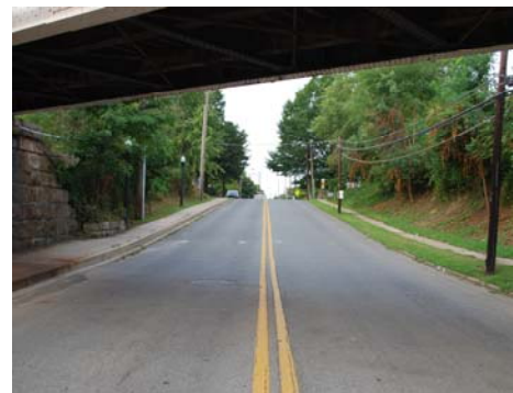
Wide travel lanes along Broad St. near Perryville Train Station.
