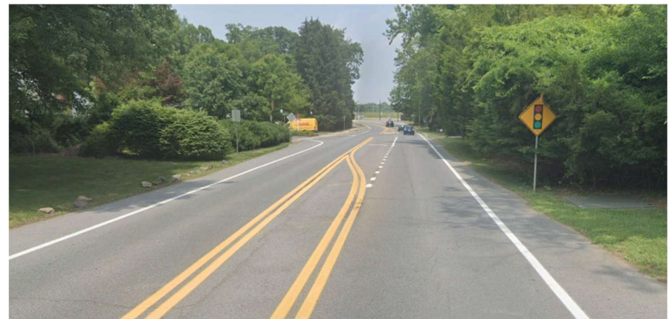
Figure 14. ACO looking north showing the Edgewood Road intersection. Source: Google Earth
