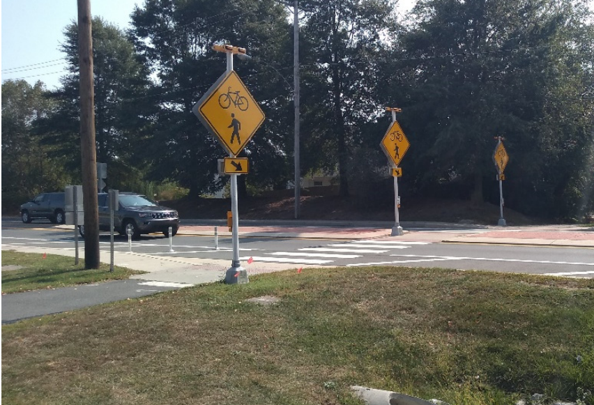
Rectangular Rapid Flashing Beacon
