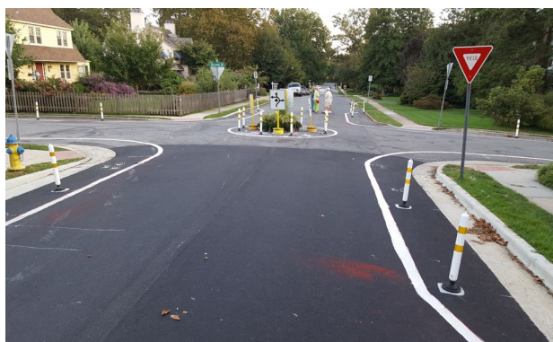
Orchard Road Mini-circle demonstration project. A mini-circle is a small raised or painted island at an intersection, designed to slow down traffic and reduce crashes in residential areas by forcing drivers to yield and navigate at lower speeds.
