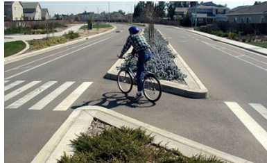
Median refuge island
