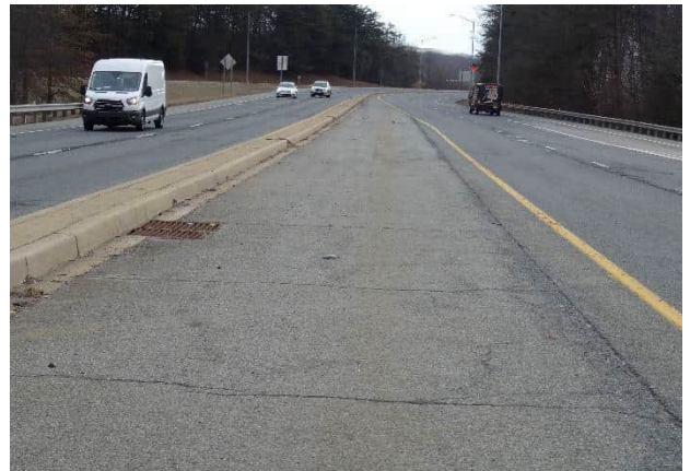
Figure 5.8: Inside Shoulder Along MD 272
