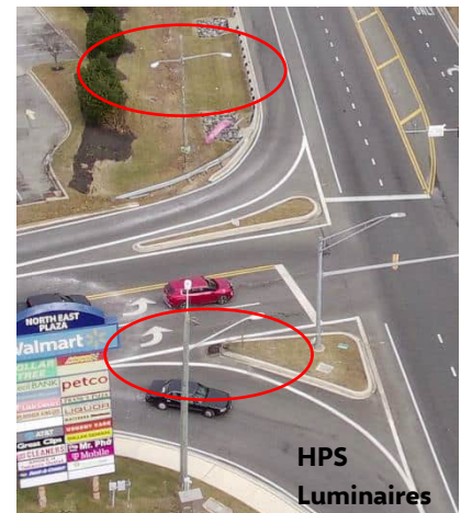
Figure 5.13: HPS Luminaires at NW and SW Corners
